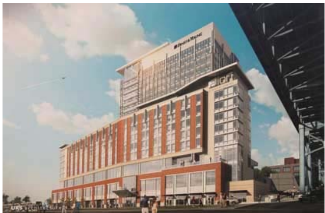
Opened this Spring, the Flats East Bank project includes a 23-story, 500,000 sq. ft.
